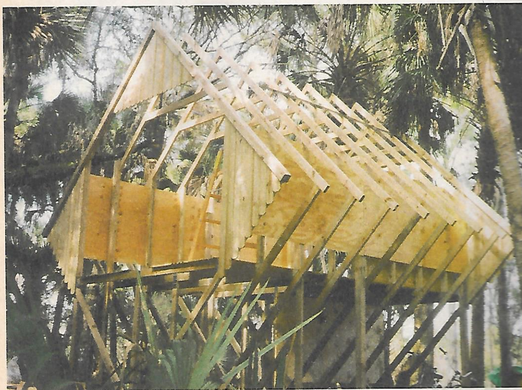
All trusses in place. This photo shows the structural importance of the center 2x4 floor support. The 4x8 plywood sheets fastened to the frame are not only an inexpensive outer wall but also add strength.
